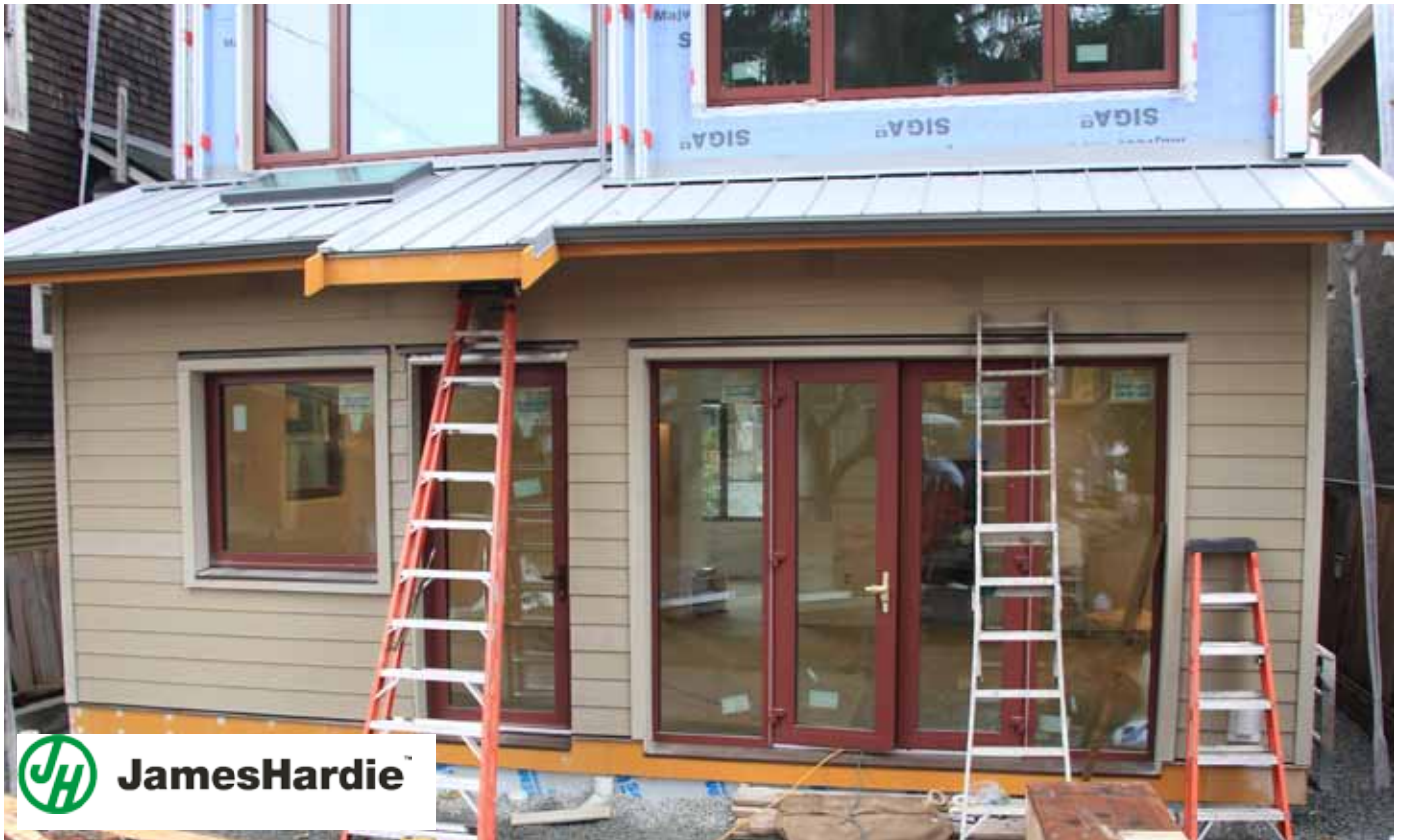
The split wall assembly required careful attention to detail around flashing, trim, corners and windows.
