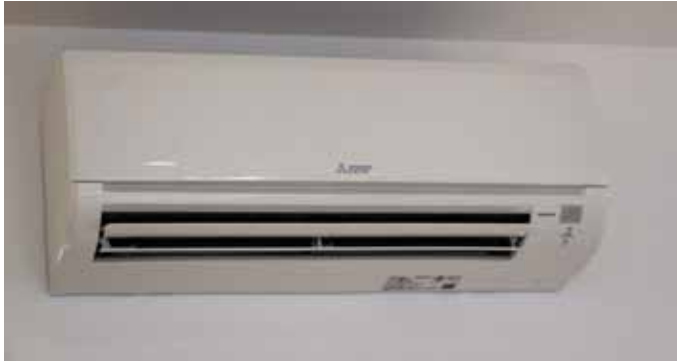
Wall mounted indoor unit to distribute heat.
