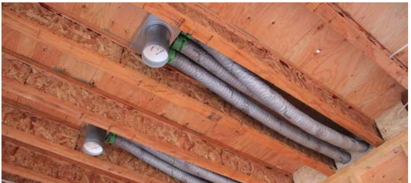
Air supply ducts from the HRV to the Living Room.
