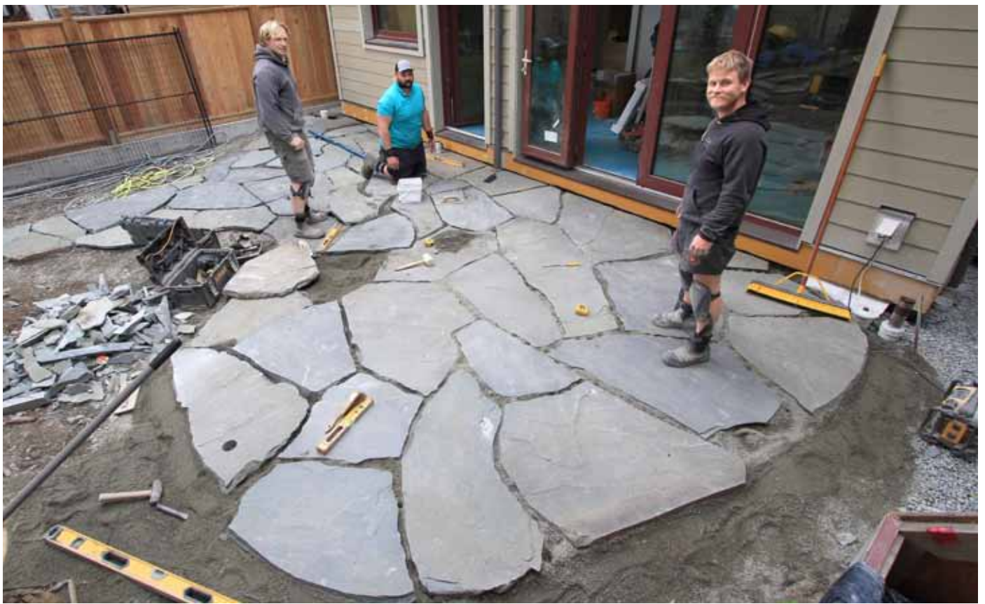
Celtic Stone installing a flagstone patio at the back of the house. The front, side and rear walkways were also constructed of flagstone.
