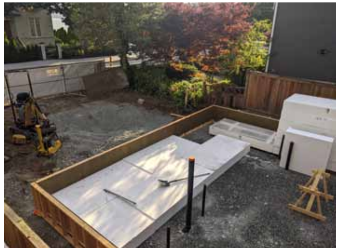
12" EPS rigid insulation Geospan.
