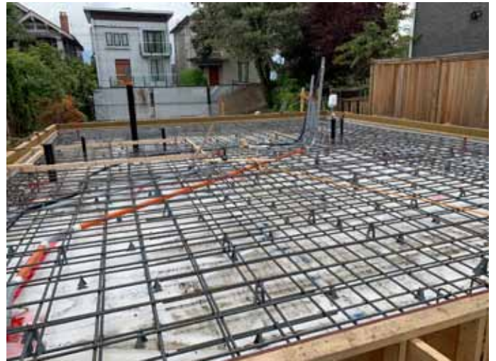
Steel rebar reinforcing ready for concrete.
