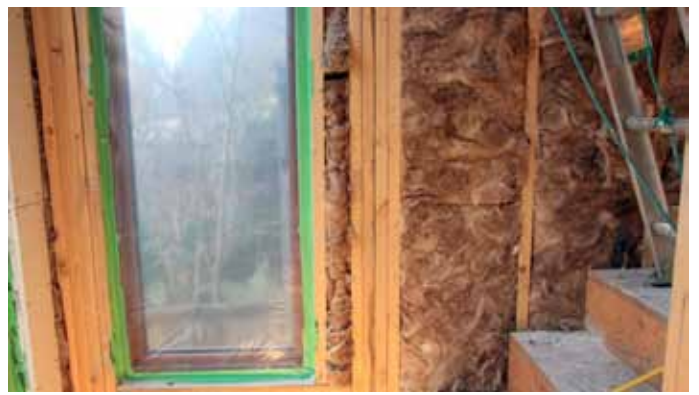
4. Fiberglass Batt insulation (filling framing cavity)
