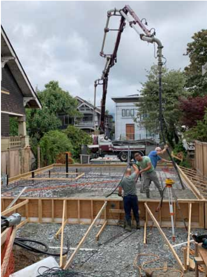
The concrete slab was poured in August 2020.
