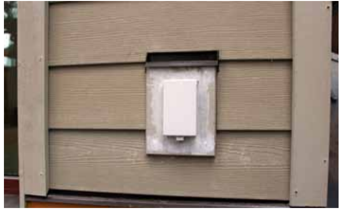
The split wall assembly required careful attention to detail around flashing, trim, corners and windows.
