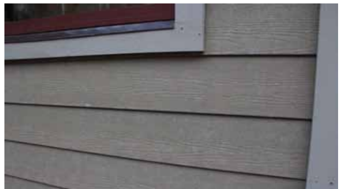
10. Hardiepanel HZ5 siding, non combustible
